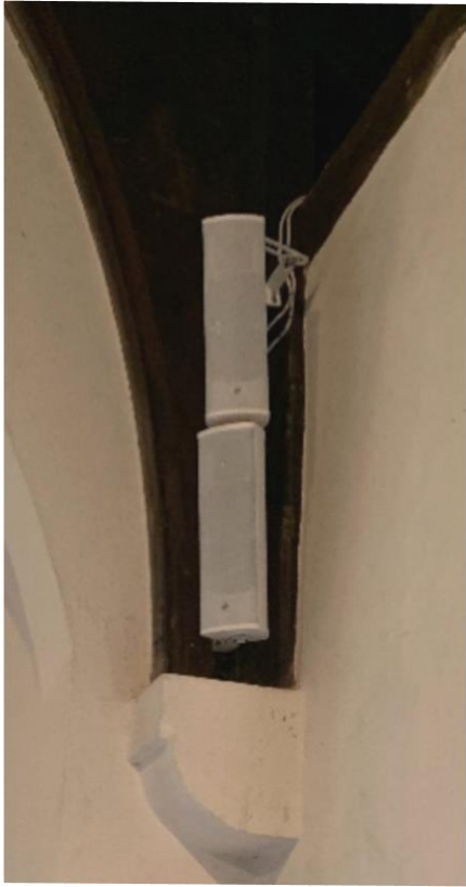
One of the Bi-Directional Sets of the wall mounted column speakers
